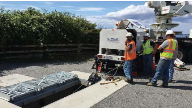
Land cable coming up at the shoreline vault after the big pull
