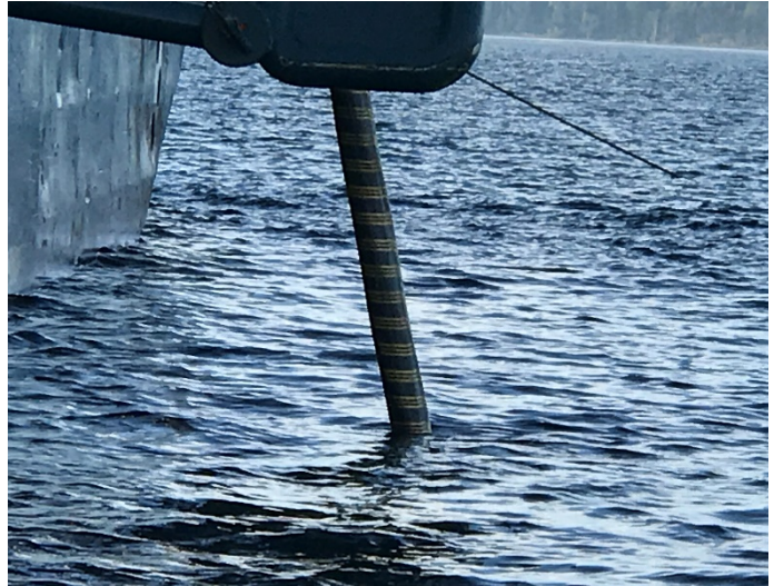
Cable Installation – Exit of Chute
