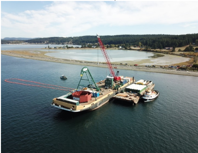
Cable Installation – Floating of cable for feed into conduit on Lopez shore
