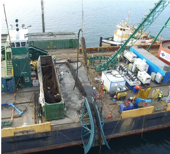
Cable Removal - Splice Canister on deck
