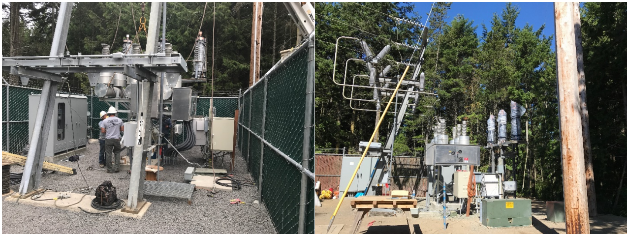
Installation of Lopez Terminal Switching Equipment
