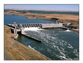
WATER IS SPILLED THROUGH THE SPILL GATES AT ICE HARBOR DAM (LEFT SIDE) FOR SAFER FISH PASSAGE WHILE GENERATING NEEDED ENERGY IN THE POWERHOUSE SIMULTANEOUSLY.
