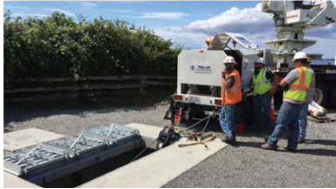
Land cable coming up at the shoreline vault after the big pull
