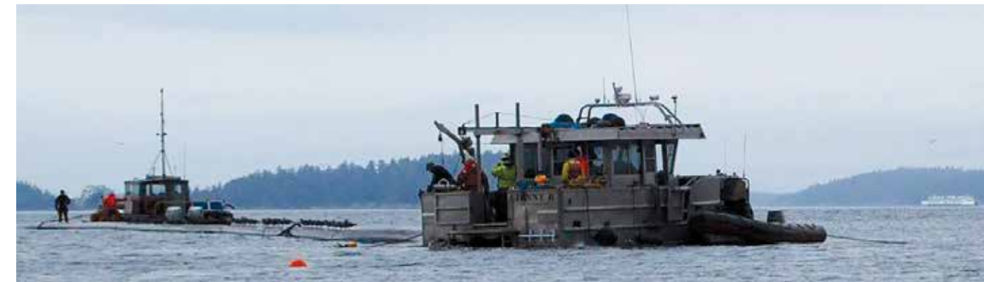
Placing the new submarine cable conduit on Lopez Island in 2015
