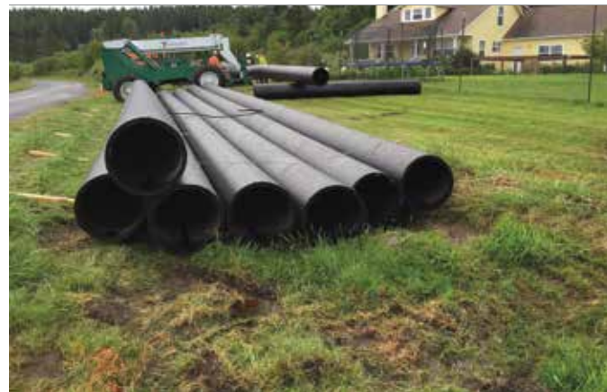
20-inch diameter conduit for land portion of the cable
